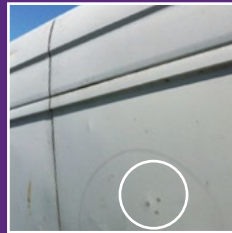
Outward dents to panel
